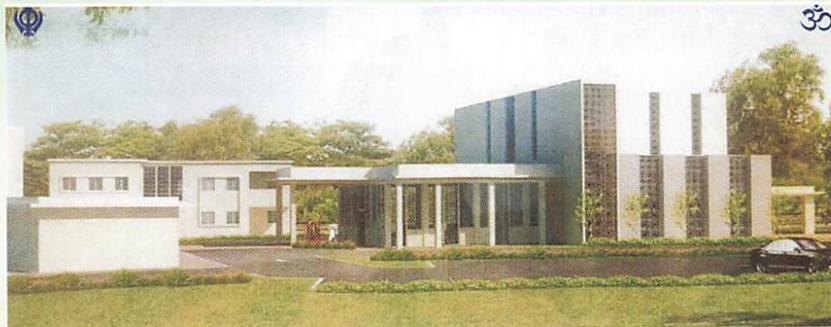
CONSTRUCTION OF SHAMSHAN BHOOMI COMPLEX AT JALAN LOKE YEW, KUALA LUMPUR
